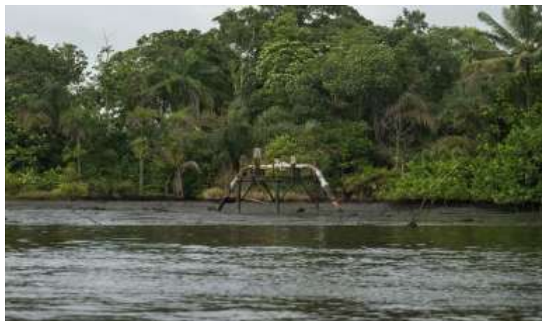
Figure (1c): Oil leak from a flow station in Bayelsa State
